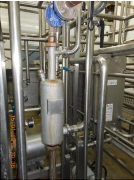
Figure 9. Milk pasteuriser with steam injection
